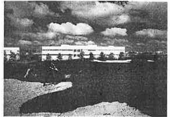
Stockley Business Park, London Borough of Hillingdon High quality buildings and landscape with recreation opportunities.
