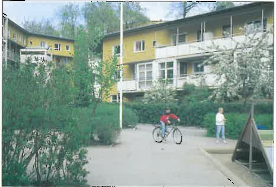
A housing cooperative is jointly owned by the residents. (Photo: JDM)
