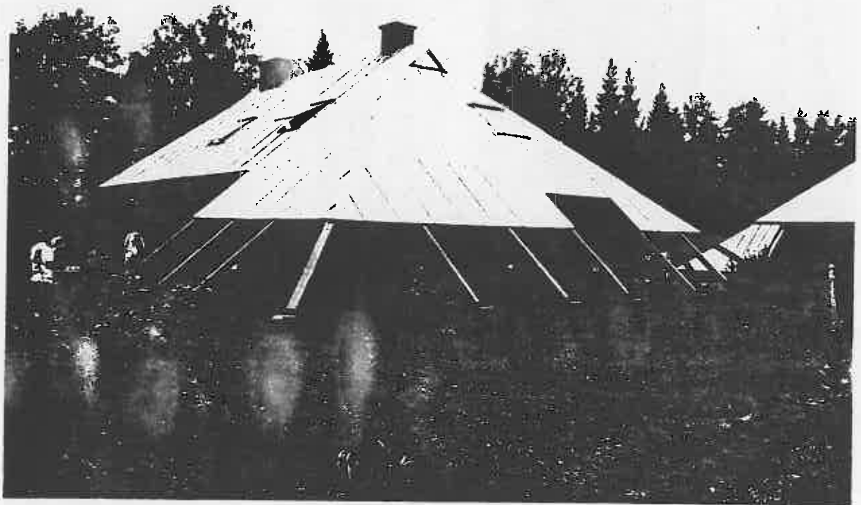
The private house in the country designed in regional traditions. 1992, arch. A. Heinrichsons, J. Dripe.
