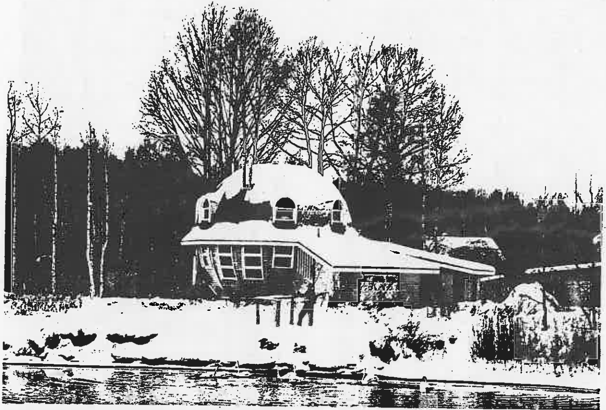
The private house designed taking into consideration the economy of energetic resources. 1996, arch. J. Bērziņš
