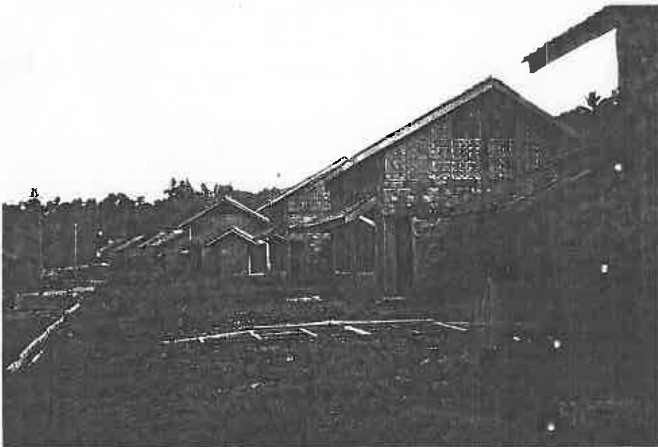
the first batch of low cost houses, ready in September, 1995
