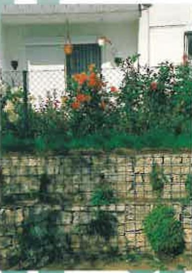
Recyclable construction materials. The chunks of broken-up concrete surfaces are smashed. They are a low-priced material that can easily be layered into edgy walls and subsequently planted.
