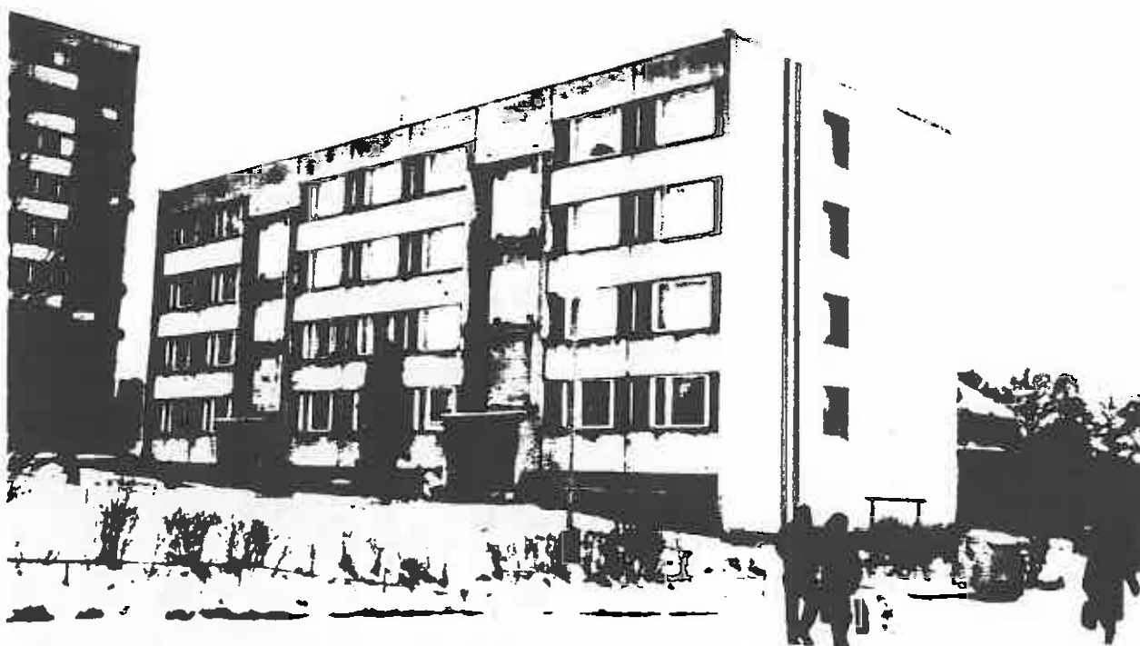
Typical prefab large-panel residential building of the seventies
